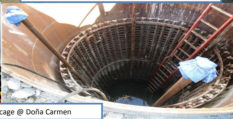
Positioning of steel casing @ Doña Carmen
